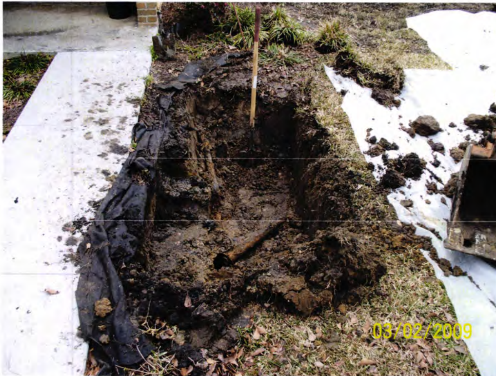
Picture 3: UST 120Banyan-2 during initial stage of removal.
