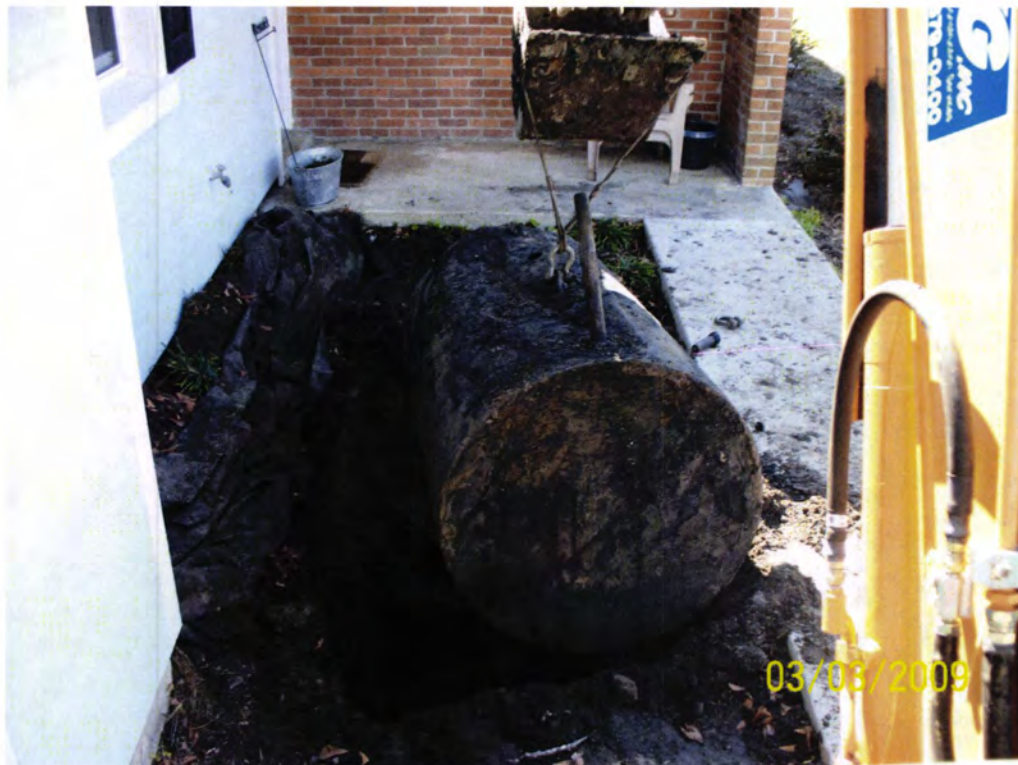
Picture 2: UST 120Banyan-1 during removal.
